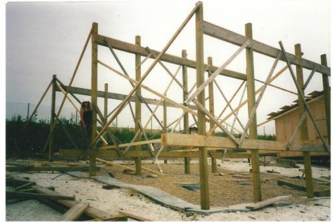
Frame going up, resting on concrete pads
